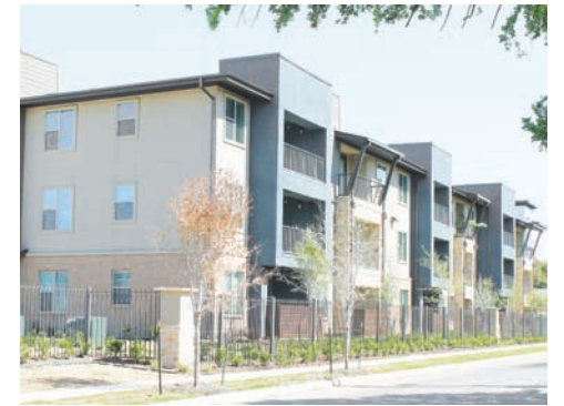
Luxury apartments are going up across the street from Cedar Springs Place. (David Taffet/Dallas Voice.)
