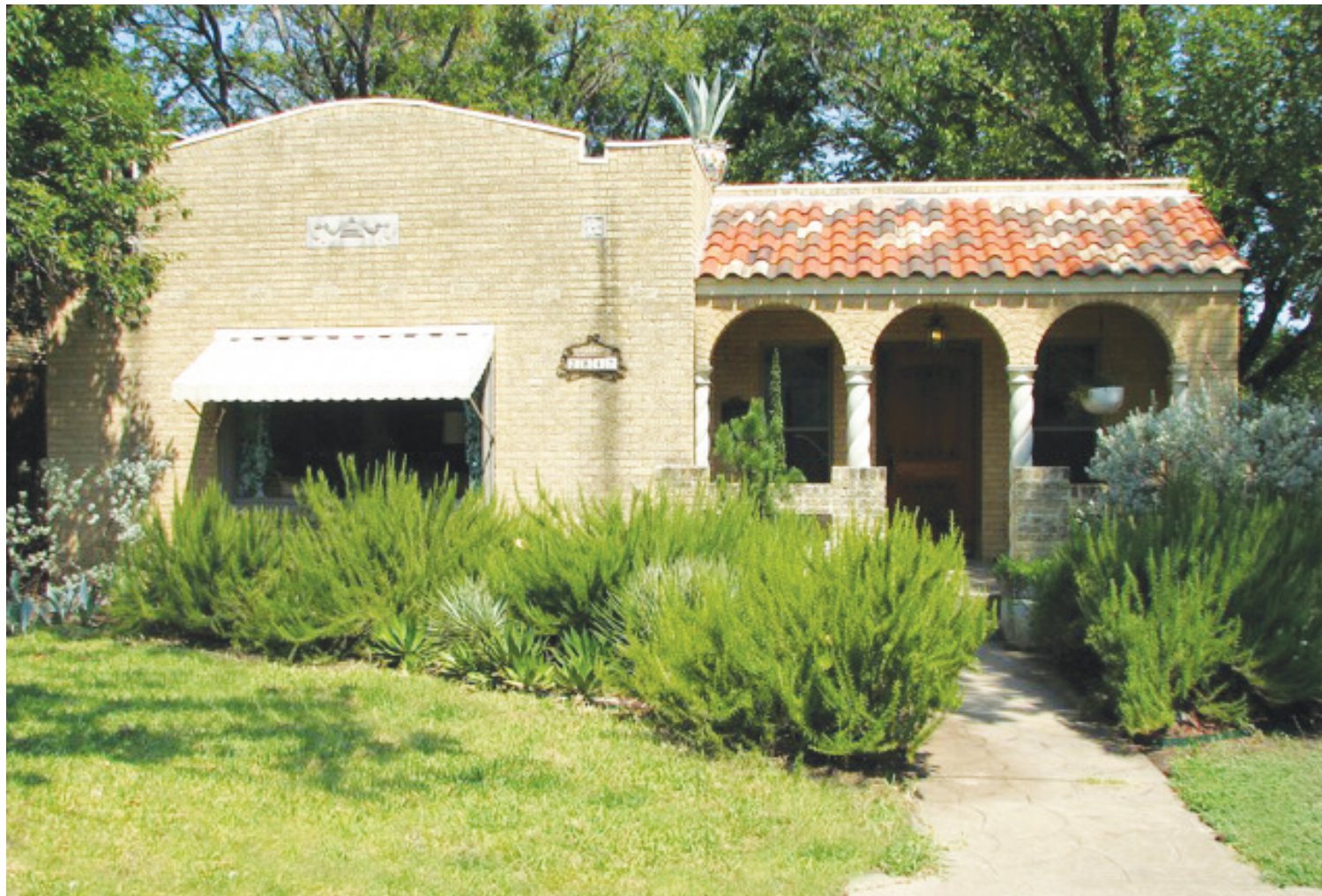
HOME SWEET HOMO | This 1927 Spanish Eclectic home in the Dells has a flat roof with a large agave plant on top and is one of a dozen homes on the Oak Cliff fall tour, which is the oldest and gayest home tour in Dallas. (Photo courtesy of Old Oak Cliff Conservation League)
