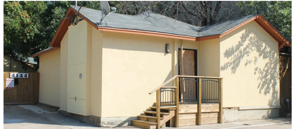
RAISING THE BAR | The new owners of the Hideaway, at 4144 Buena Vista in Uptown, have extensively remodeled it since the iconic gay bar closed in 2009. (David Taffet/Dallas Voice)
