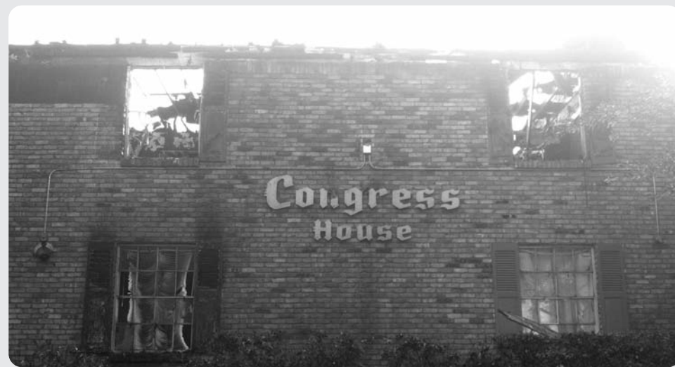
GUTTED | Dallas firefighters battled a three-alarm blaze Wednesday morning at the Congress House Apartments at 4320 Congress Ave. that destroyed 10 apartments. (Anna Waugh/Dallas Voice)
